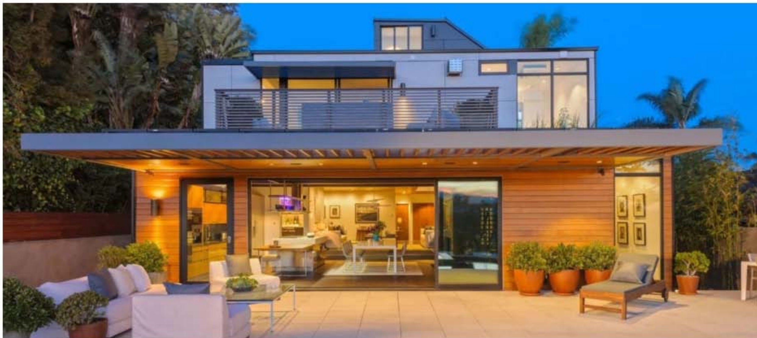
Photo courtesy of Plant Prefab
